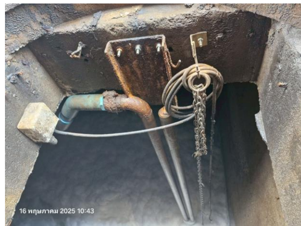
Equalizing Tank (EQ)
